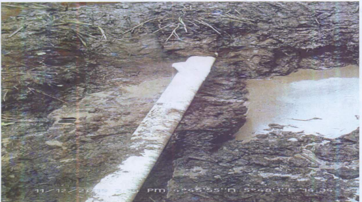
FIG.2: SHOWING THE PIPELINE AFTER REPAIRS
