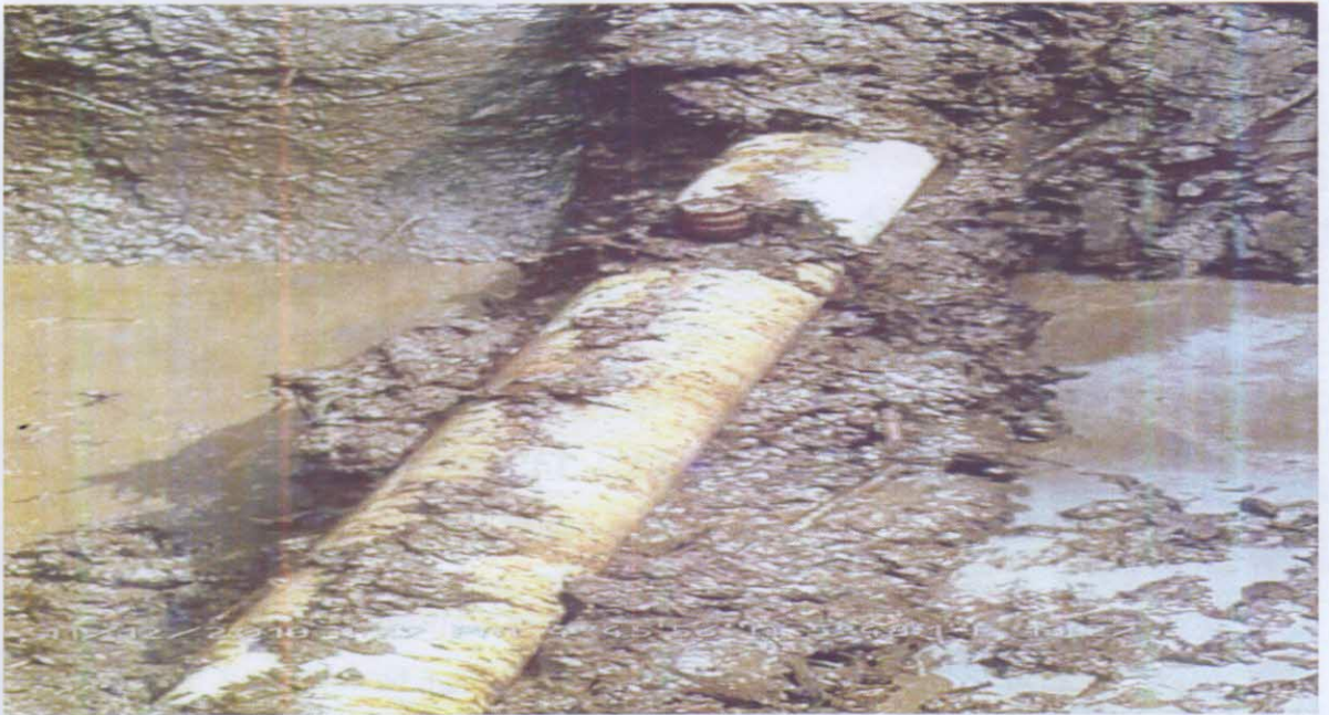
FIG. 1: SHOWING THE INSTALLED 2" VALVE BEFORE REPAIR WORK
